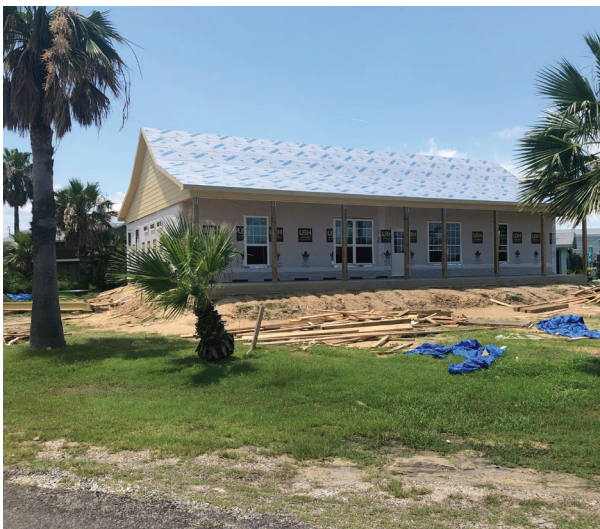
A home under construction in Copano Cove.
